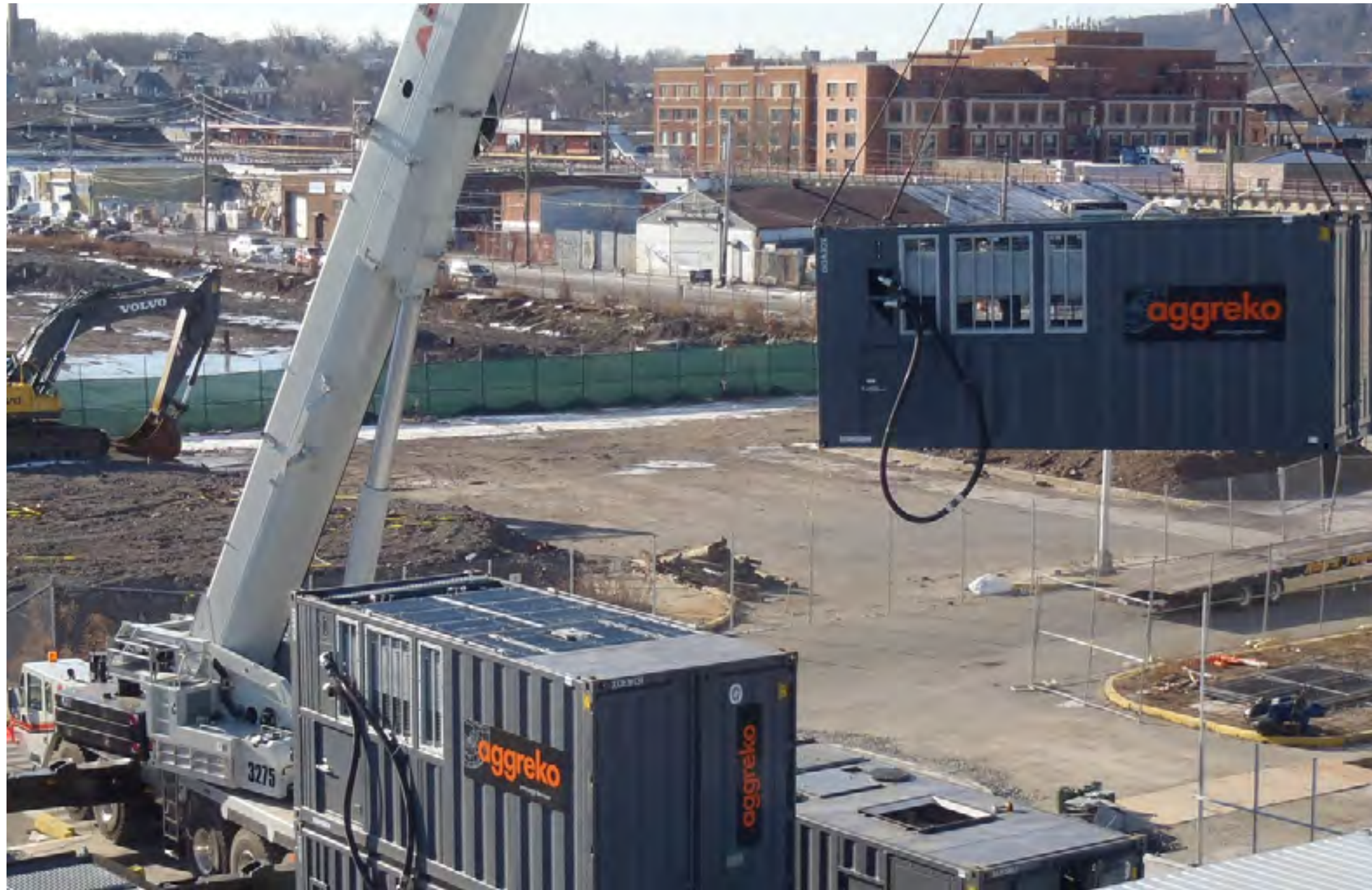
Container generator being craned into place at data centre construction site.
