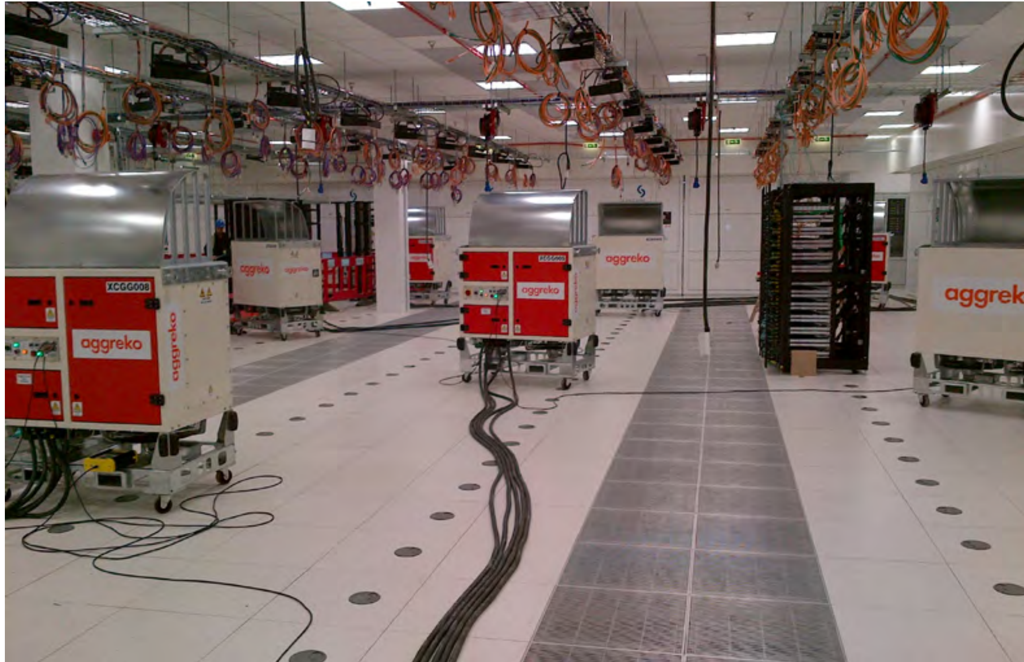
4 MW heat load test using loadbanks.
