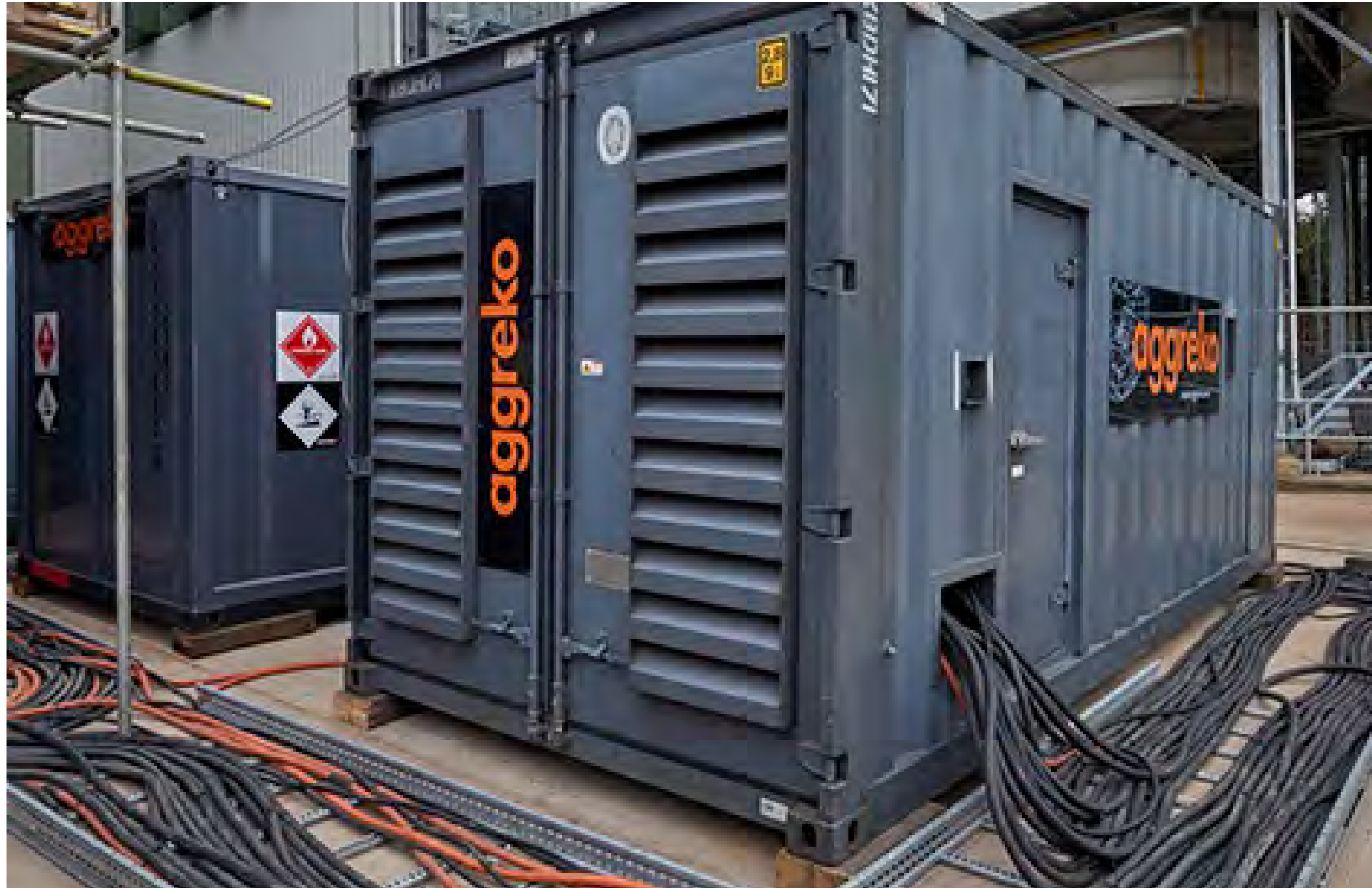
Site acceptance testing using loadbanks to test site generators.
